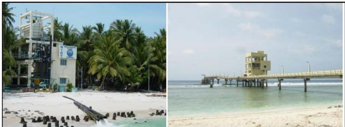
Fig 7: Low Temperature Thermal Desalination ( LTTD) plants in Lakshadweep set up by NIOT at Kavaratti, and Agatti
